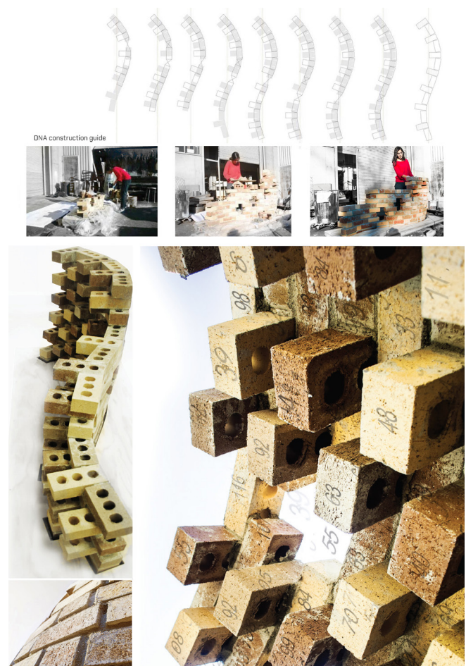
Figure 3: The paper guides and the process of building a full-scale prototype
