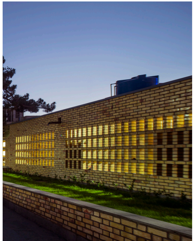
Figure 1. Figure 1: Brick screen wall at the Gohar Khatoon school project . Image credit: Nic Lehoux
